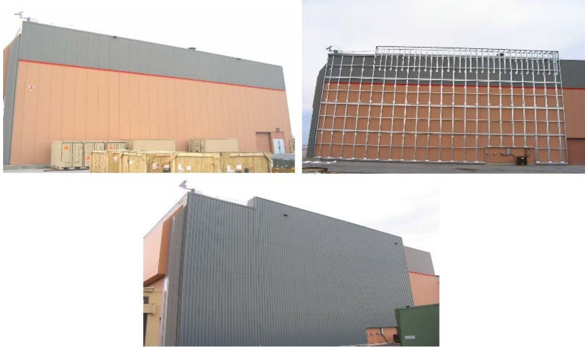
Figure 9: Picture of UTC Wall - Before, During, and After Installation (Source: Rowley, 2006)
