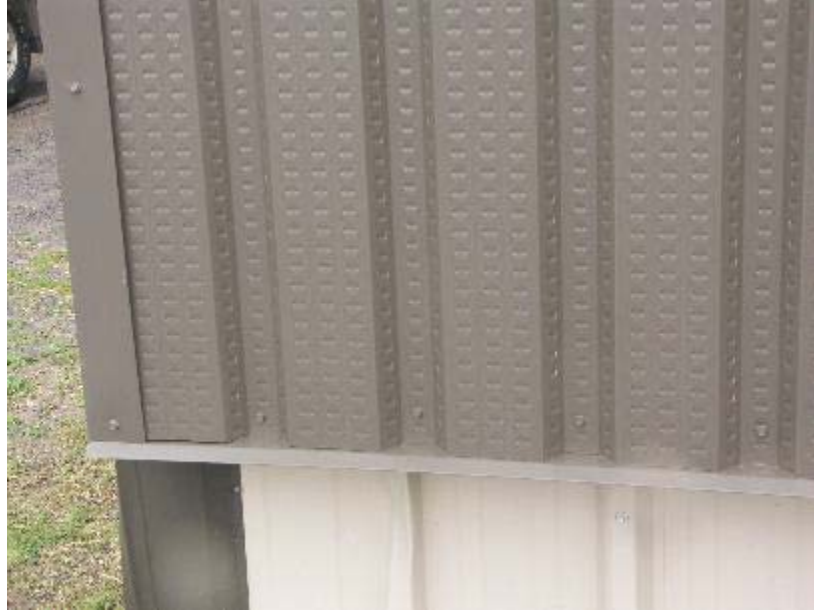
Figure 11: Surface of a Typical Corrugated UTC Wall
