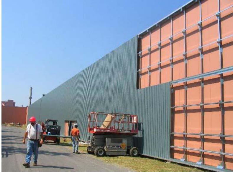
Figure 16: Installation of UTC at Fort Drum, NY (Source: SolarWall® - Fort Drum, 2008)
